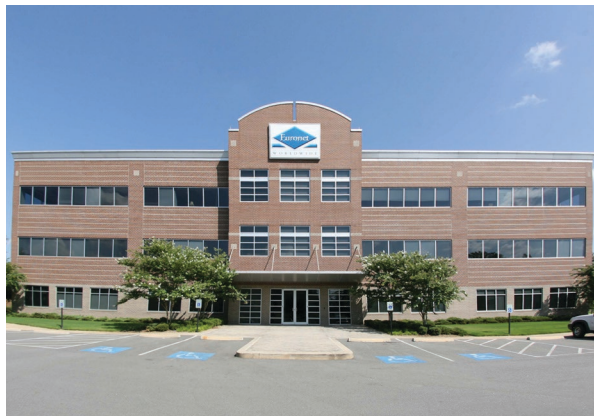
Euronet Worldwide Bldg | 17300 Chenal Pkwy ±2,052 – ±4,275 SF OFFICE SPACE FOR LEASE
