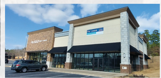
City Silo Table + Pantry and vacant space.
